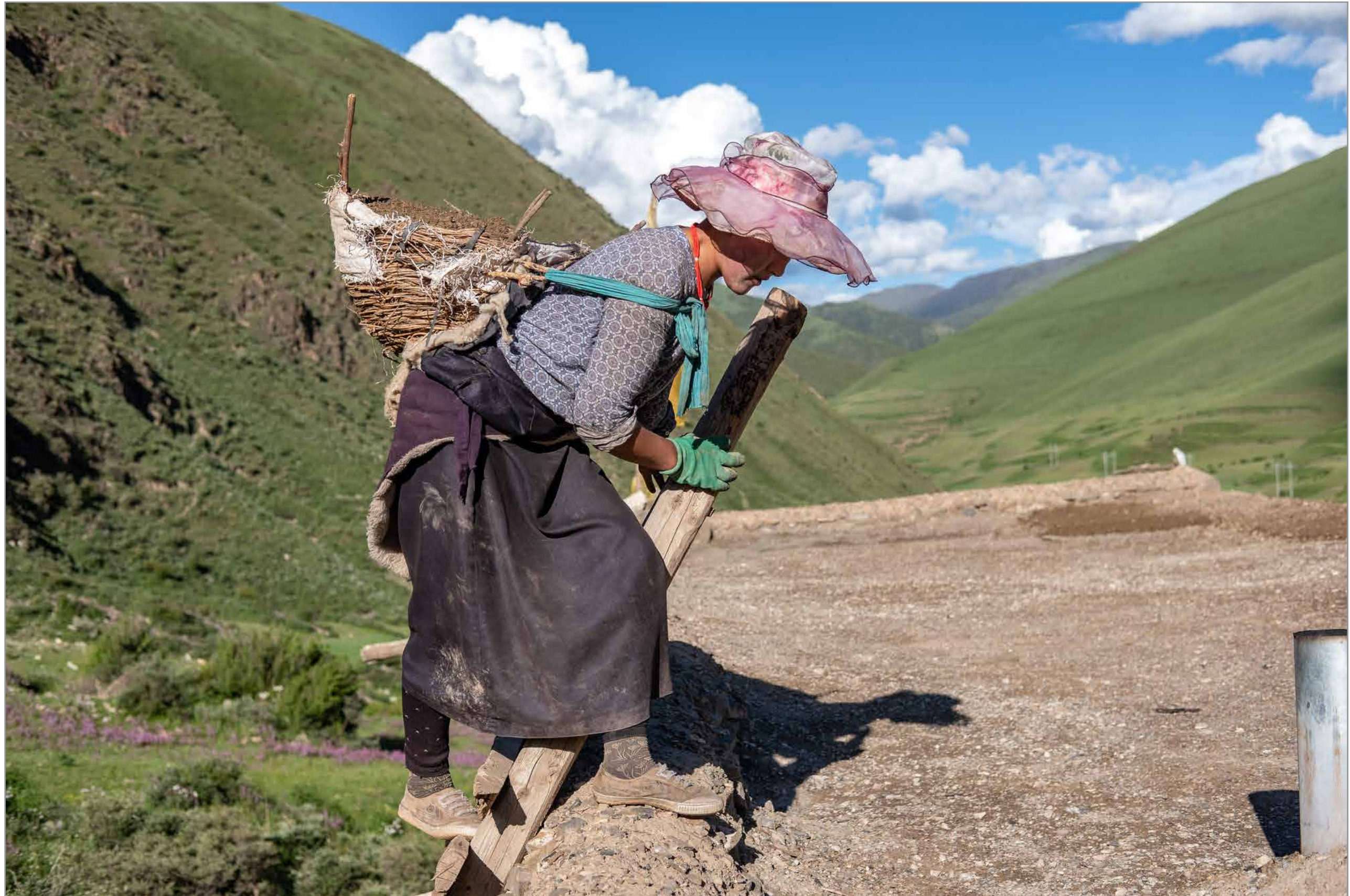
Jamyang Tsomo carries a handwoven basket filled with dirt up to the roof of her family's home. After she has removed weeds and stones from the roof, she fills the dips and holes to prevent water leaks or collapse. Besides her mother, Jamyang Tsomo is the only woman in the household, and is responsible for most of the domestic duties.
